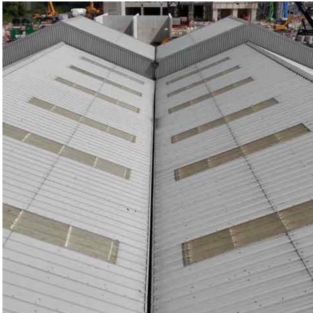
Photo 7 Roof 1 Roof covering and Rooflights
